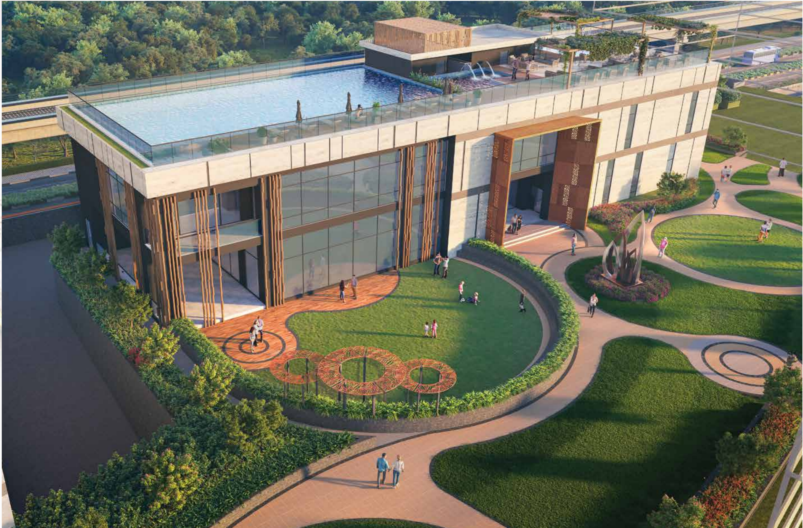
Artist's impression and not actual site image. This is for representational purposes, indicating the amenity / development and not the actual delivery.
